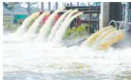
Polluted sewerage water Water pollution
