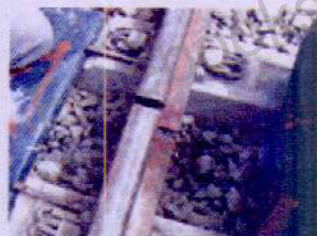
Figure 8.15: Gaps are left in railway tracks to compensate thermal expansion during hot season.
