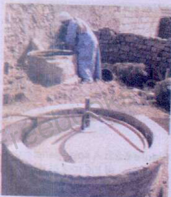
Figure 6.26: A biomass plant using animal dung
